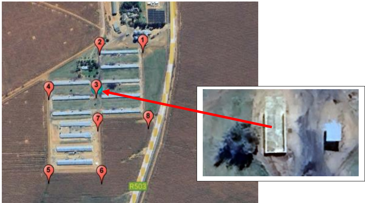
The chicken houses of the WeeBee Boerdery operation with the incinerator unit to be installed in the middle as indicated. [Cemented area of ± 84m 2 ]
