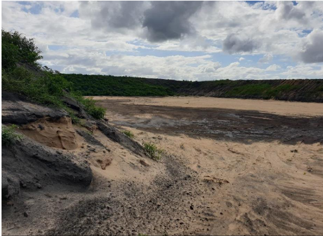
Figure 7: Smuts storage dam. Decommissioned dam made accessible to farmers
