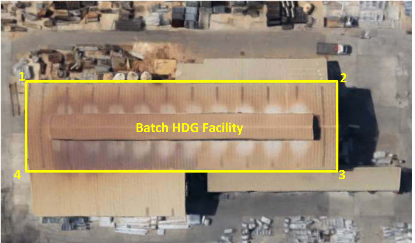
Hot Dip Galvanizing Facilities GPS Co-ordinates (DMS Format)
