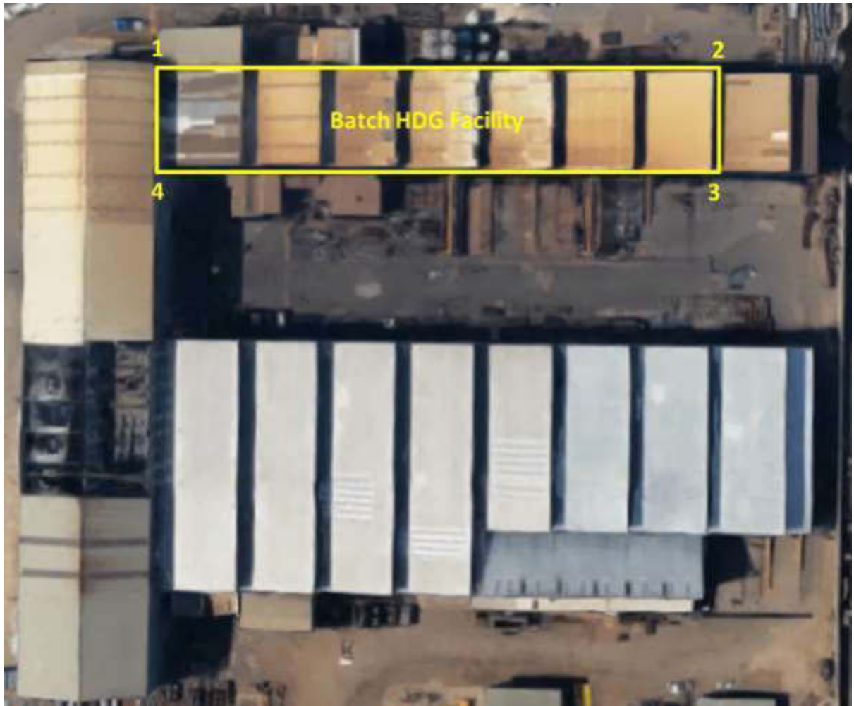
Hot Dip Galvanizing Facilities GPS Co-ordinates (DMS Format)
