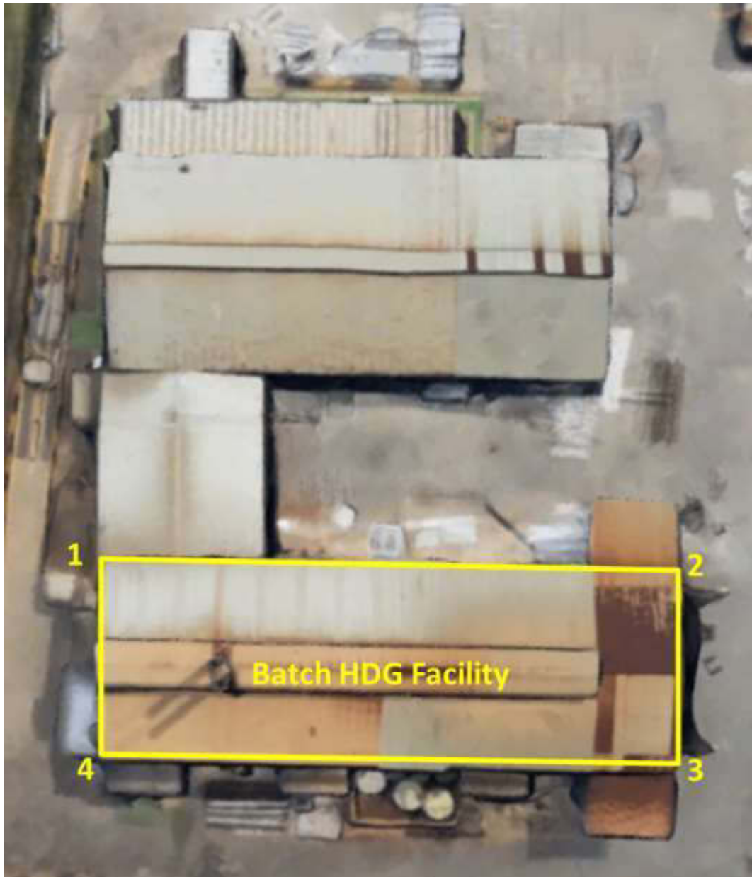
Hot Dip Galvanizing Facilities GPS Co-ordinates (DMS Format)
