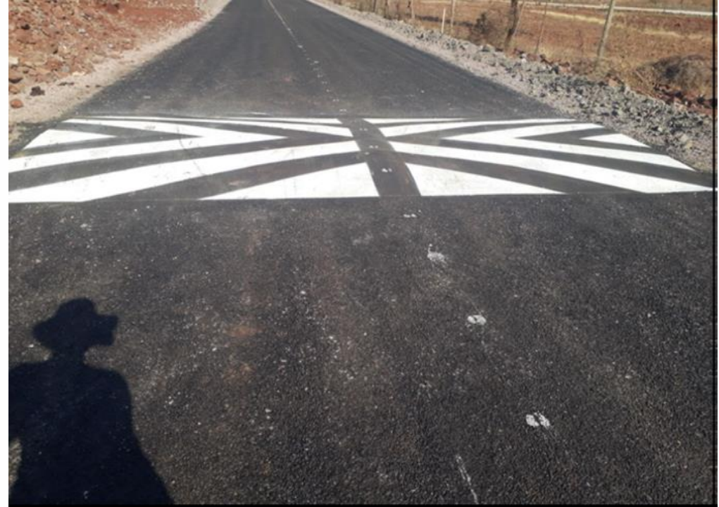
After: Asbestos free road at Ga-Mafefe
