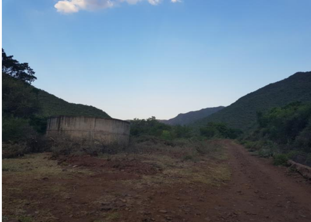
Before: Gravel road at Ga-Mafefe Mafefe
