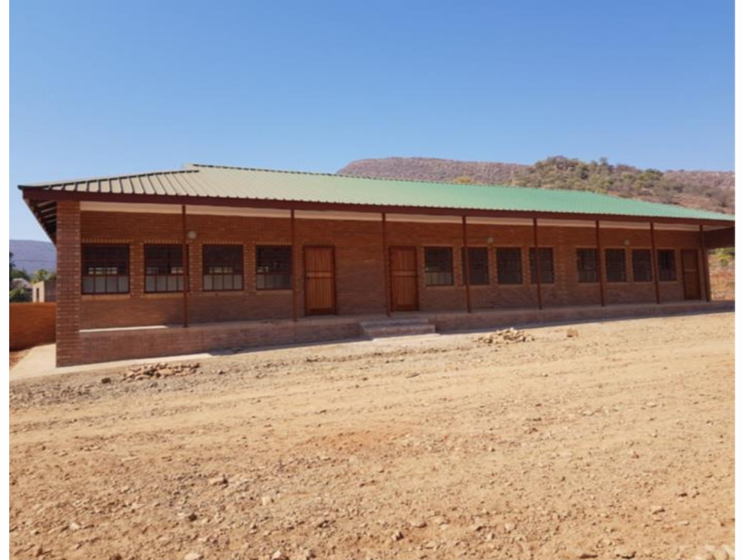
After: Asbestos free classrooms at Ga-Mafefe
